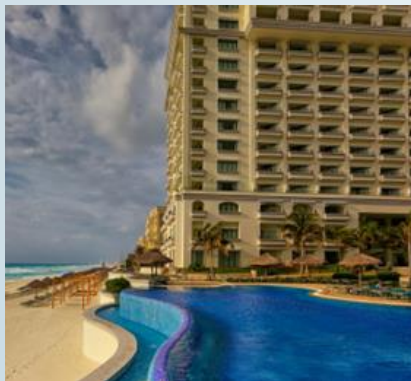
Commercial Development Pollution, runoff & increased volume
